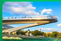
Floating Bridge Moscow
